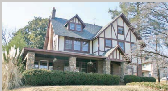
Articulated facade: note it is a composition of small forms.
