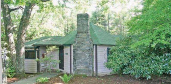
Oversized chimney typical of a Highland Resort structure.
