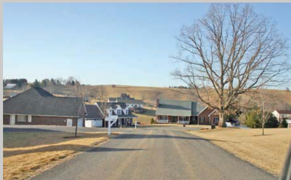
Prime and seal road for moderate use.
