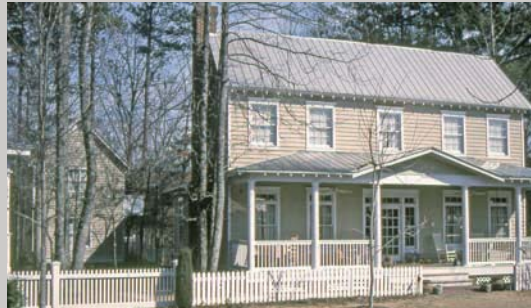
Recent example of porch and fence detail.
