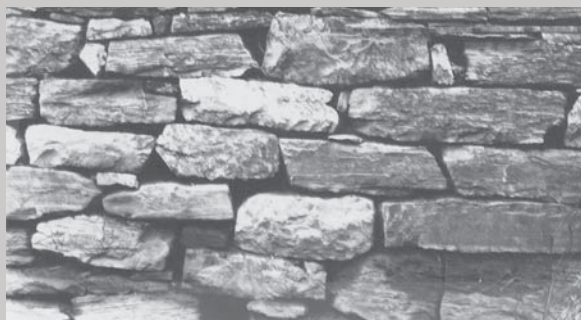
Local house foundation that served as a model for Parkway masonry. (Edward H. Abbeuhl, 1935. Blue Ridge Parkway Photographic Archives.)
