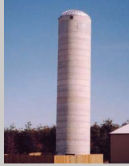
Grain silo cellular tower. (Sollenberger Silos, LLC.)
