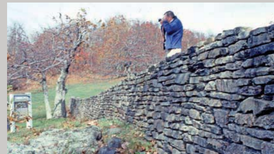
Exposed ledgerrock wall at Rocky Knob. Notice batter on wall.
