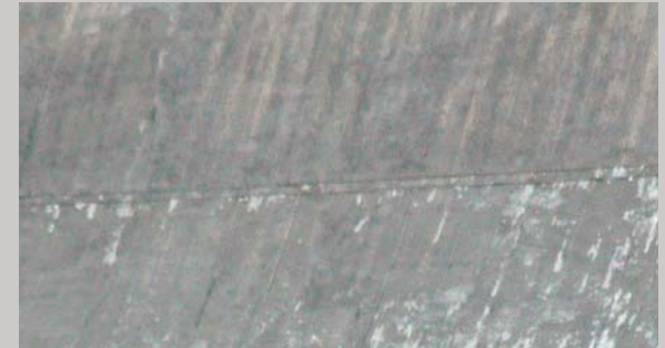
Metal roof showing aged patina.
