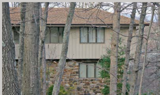
Vertical casement windows.
