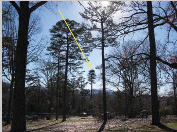
Tree cell tower can be used in wooded areas. This one is near the Folk Art Center along the Parkway in Asheville (J. David Anderson.)
