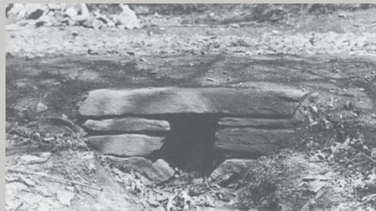
Culvert headwall. (Edward H. Abbeuhl, 1937. Blue Ridge Parkway Photographic Archives.)
