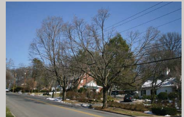
Some power companies use "tree cable" in special-request areas. Tree cable costs more to install, but tree limbs can grow very close to the electrified lines.
