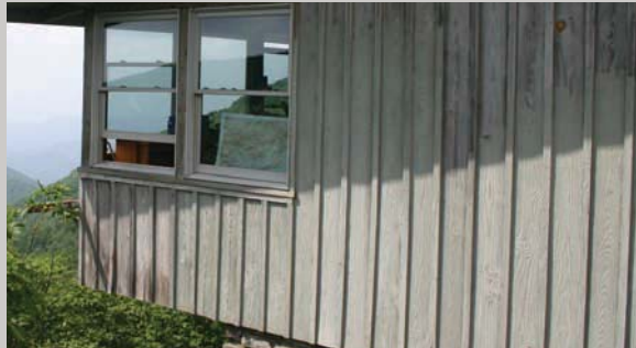
Board and batten siding.
