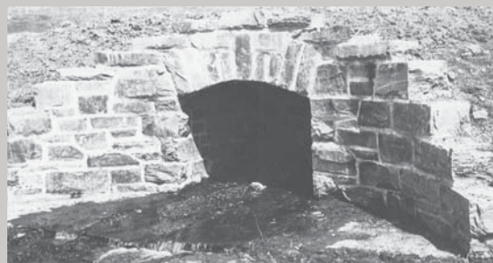
Box culvert wingwall. (George Wickstead, 1936. Blue Ridge Parkway Photographic Archives.)
