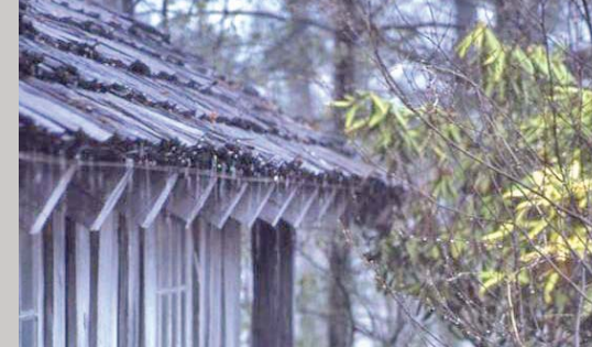
Brackets and extended eaves.
