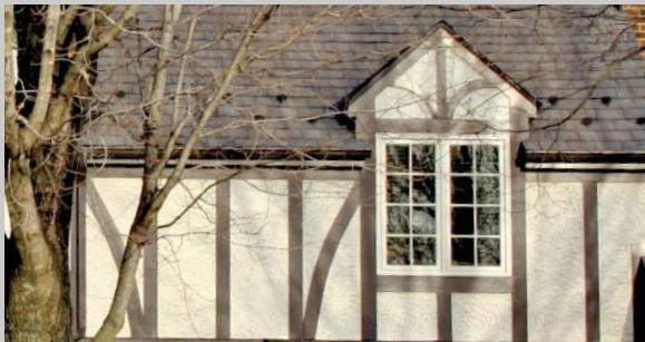
Windows break up vertical mass.
