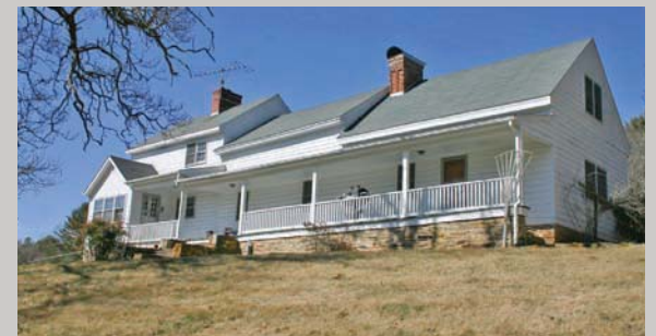
Stone foundation walls.
