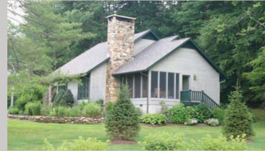
Clean roof forms.
