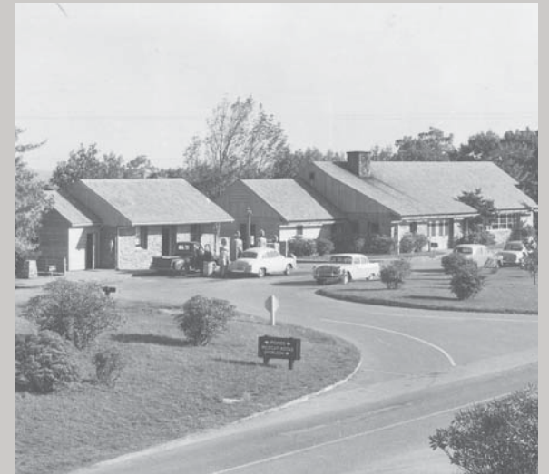
Architect Edward Abbeuhl's Bluffs Coffee Shop, seen here in 1956, bears a striking resemblance to the vernacular mass, shape and scale seen in Hall's barn photograph above. (Blue Ridge Parkway Photographic Archives.)
