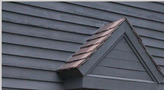
Clapboard wood siding.
