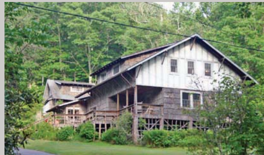
Second story shelters the porches.
