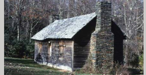
Early experiments in vernacular design were used on this CCC camp structure built near Rocky Knob. This building exhibits a native stone chimney, clapboard siding, and a shake roof.
