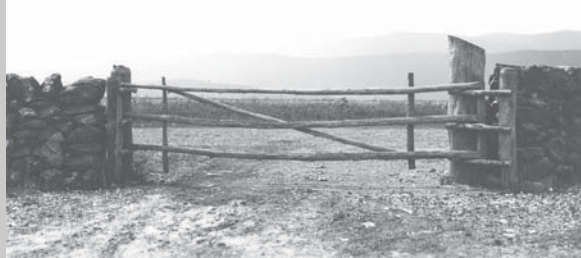
Wood pole gate between field stone fence. (Wally A. Johnson, 1943. Blue Ridge Parkway Photographic Archives.)
