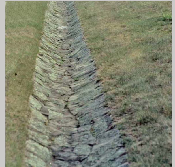
Typical stone gutter.
