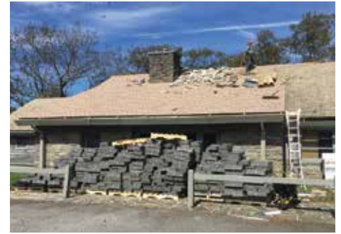
From the Top: Roof work begins at Bluffs
